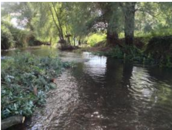
Completed job: deflector on the left, scouring logs on the riffle, and faggots against the right bank (Image © Mike Blackmore)
